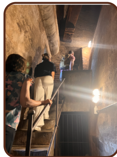
The stairs between the inner and outer shells of the dome
